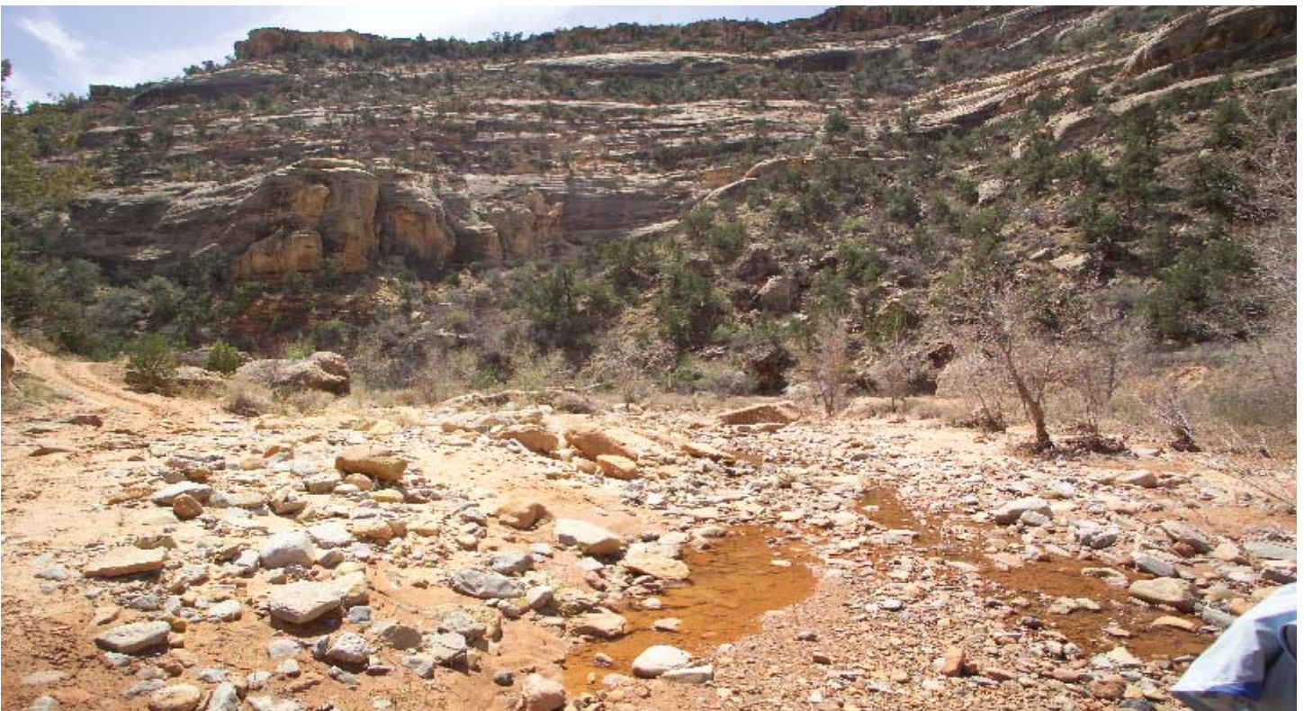
FIGURE 6. Downstream view of Figure 4 where 4-wheel drive route crosses the channel. Channel is in Non-Functional condition due to loss of bank, soil and vegetation. Arch Canyon, San Juan County, Utah.
