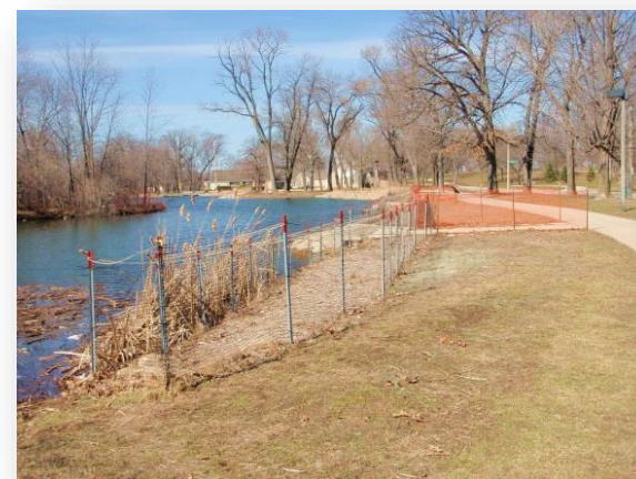
Temporary fencing to protect a park shoreline and newly-planted goose-resistant vegetation from wear and tear by geese
