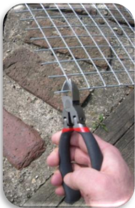
Using a wire cutter to trim welded wire mesh
