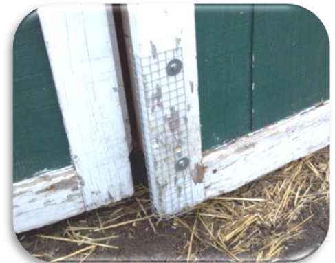
Hardware cloth applied to a door-edge to keep animals from gnawing on it
